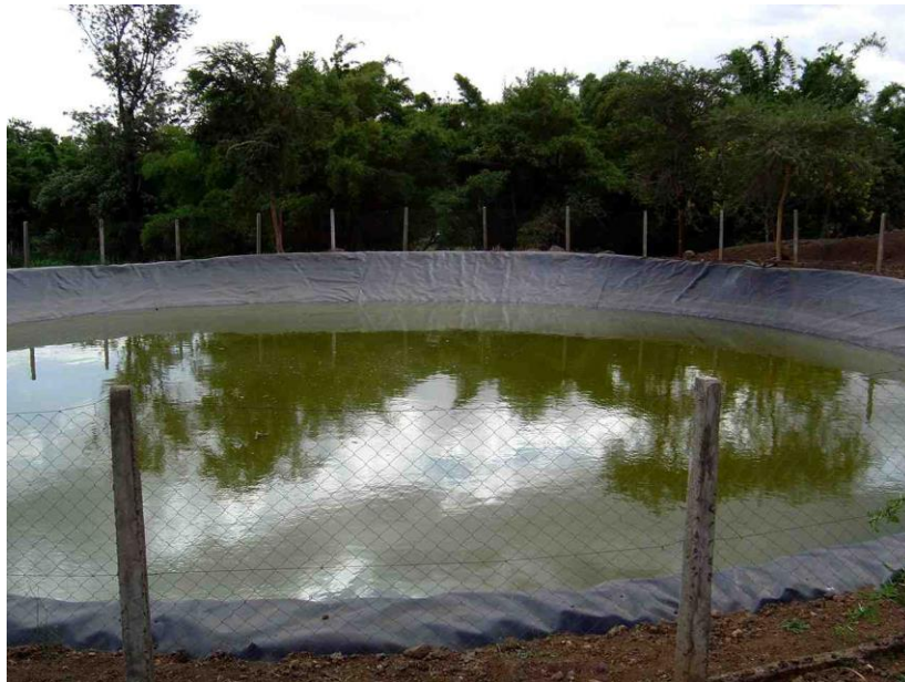
Figure 16. Lined pond, Arusha 2006. Information should be collected on cost-benefit of these.
